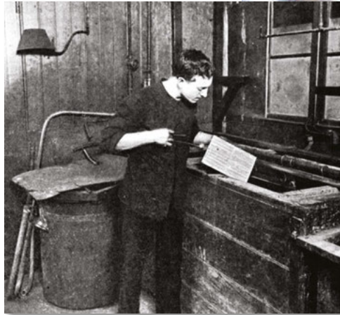
Fig 10 Aside from it being a plate instead of a cylinder, little has changed in more than 100 years. The modern-day baths at Saueressig would be instantly recognisable to the young man in this 1913 photo
